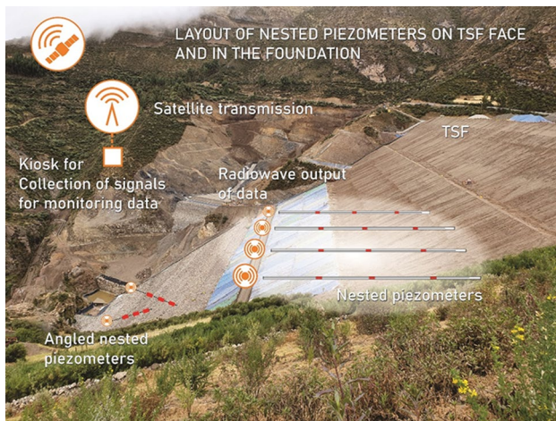
Fig. 10 Nested piezometers installed in a TSF face and foundation
